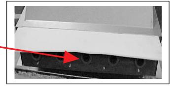
Lift the installation to allow the main head to be installed. When head is placed into position, release the insulation; it will now shield the high limits from the heat produced by the flue collector.
