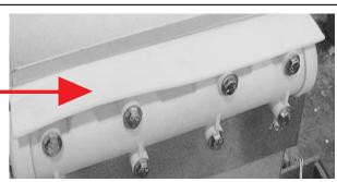
Return head removed and new tube seals installed. Now ready to accept the installation of the main head.
