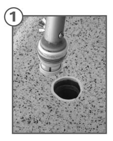
Use removal tool made for existing nozzle to remove one nozzle at a time by rotation 1/4 turn counter clockwise to unlock. The system is hydraulically balanced, so the same size nozzle needs to go back into the appropriate hole.
