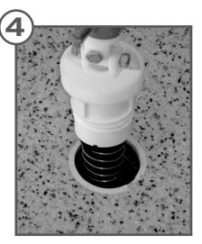
Press the top of the complete RetroJet nozzle onto the three prongs of the RetroJet installation tool\*. Guide the nozzle into the hole in the pool floor and then rotate clockwise 1/4 turn to lock in place.
