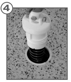
Press the top of the complete RetroJet nozzle onto the three prongs of the RetroJet installation tool\*. Guide the nozzle into the hole in the pool floor and then rotate clockwise 1/4 turn to lock in place.
